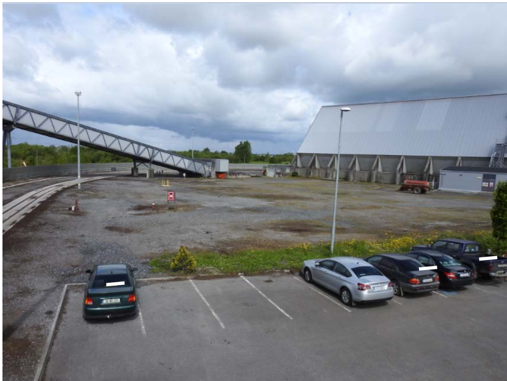
Figure 4-8: Ground view of Biomass Storage Slab A
